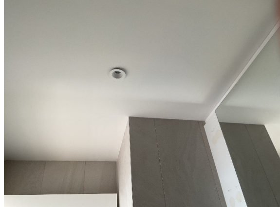
12445 - 2 - CEILING~PAINT ON POT LIGHT, OTHER POT LIGHT NOT FLUSH TO CEILING
