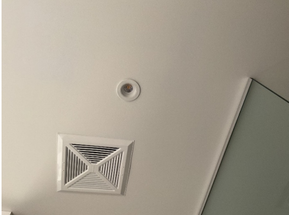
12445 - 1 - CEILING~PAINT ON POT LIGHT, OTHER POT LIGHT NOT FLUSH TO CEILING
