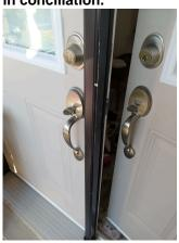
78227 - 2 - IMG\_20230828\_114421 - Front door astragal is damaged need replaced. This house is in conciliation.
