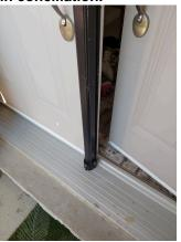
78227 - 3 - IMG\_20230828\_114423 - Front door astragal is damaged need replaced. This house is in conciliation.
