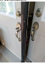
78227 - 4 - IMG\_20230828\_114425 - Front door astragal is damaged need replaced. This house is in conciliation.
