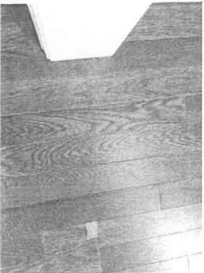
147323 - 1 - FLOORING~CHIP ON 7TH PLANK FROM LEFT ARCH BY MUD ROOM DOOR PLANK
