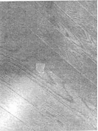
147322 - 1 - FLOORING~CHIP ON 11TH PLANK FROM LEFT INDENT WALL LEFT OF VENT
