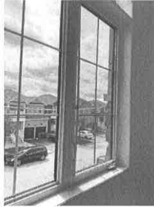
147797 - 1 - WINDOWS~WINDOW SCREEN BOWED BEDROOM RIGHT OF STAIRS
