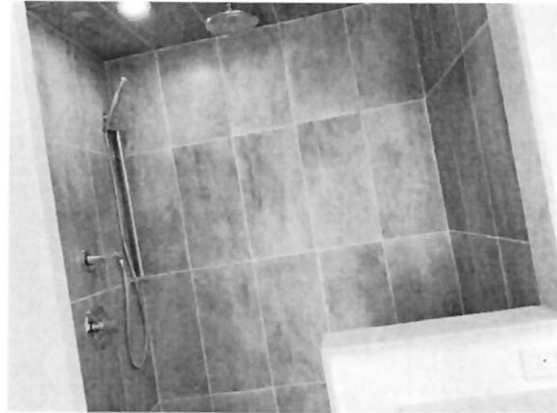
148267 - 1 - SHOWER ENCLOSURE~SHOWER GLASS NOT INSTALLED
