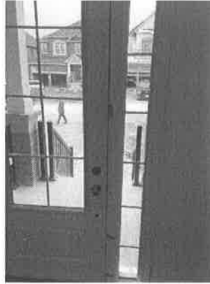
150125 - 1 - FRONT DOORS~ADJUST FRONT DOOR AND GAP AT TOP TO BOTTOM GOES THIN TO THICK
