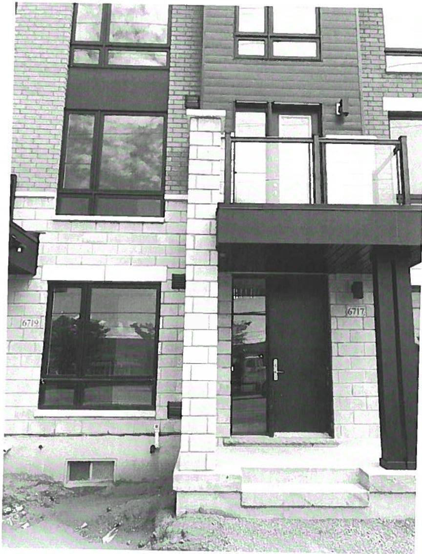
Blk#4 Unit#21 front column remove 1 course of stone:
