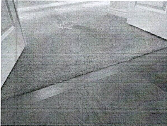
152123 - 3 - FLOORING~ADJUST CARPET SHIM AT ENTRANCED TO BATH TOO HIGH AND CARPET RAISED AT RIGHT CORNER OF WINDOW
