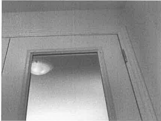
151420 - 1 - FRONT DOORS~SCREW COVERS MISSING AT FRONT DOOR
