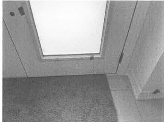
151420 - 2 - FRONT DOORS~SCREW COVERS MISSING AT FRONT DOOR
