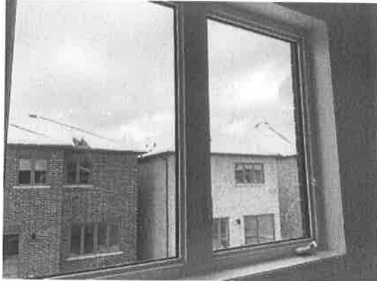
152312 - 1 - WALLS~SCREEN ON WINDOW NOT INSTALLED
