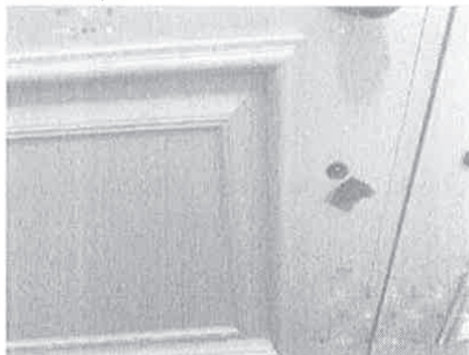
149504 - 1 - FRONT DOORS~SCREW COVER NOT INSTALLED
