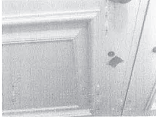
149504 - 1 - FRONT DOORS~SCREW COVER NOT INSTALLED
