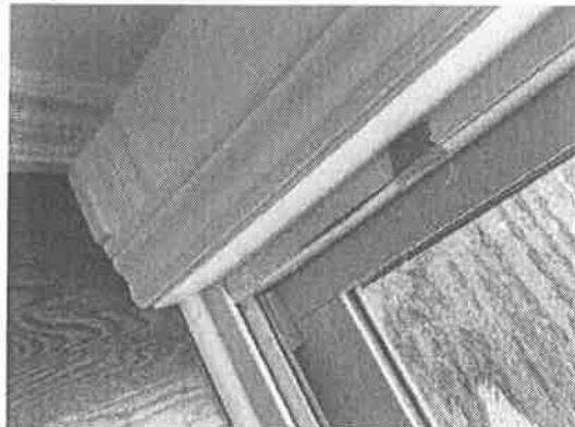
153639 - 1 - WINDOWS~BUBBLE ON LEFT MULLIN LEFT OF DOOR AT TRIM
