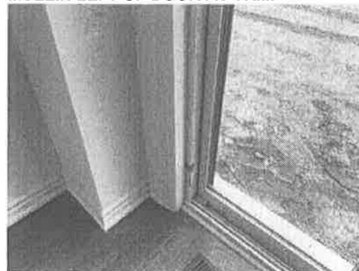
153639 - 2 - WINDOWS~BUBBLE ON LEFT MULLIN LEFT OF DOOR AT TRIM
