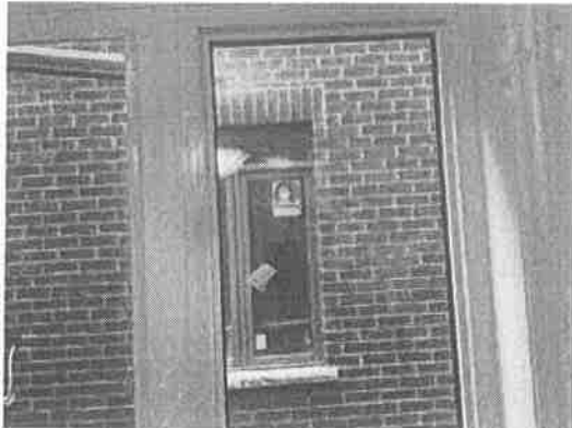
153623 - 2 - WINDOWS~SCRATCH ON RIGHT FIXED GLASS RIGHT OF OPERATING WINDOW
