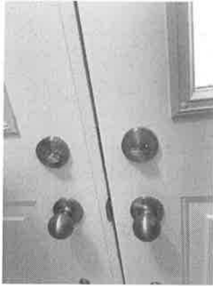
154112 - 1 - FRONT DOORS~CHIPS AT MIDDLE ASTRICAL
