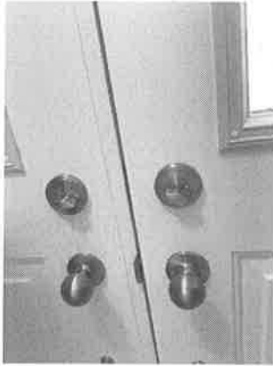
154112 - 1 - FRONT DOORS~CHIPS AT MIDDLE ASTRICAL
