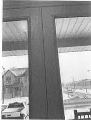
154112 - 3 - FRONT DOORS~CHIPS AT MIDDLE ASTRICAL
