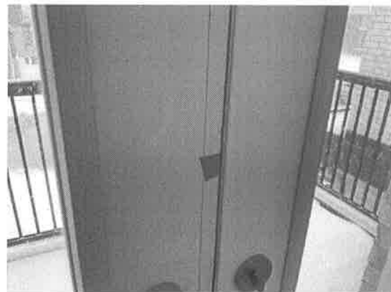
154118 - 1 - WINDOWS~DAMAGE AT ASTRICAL MIDDLE
