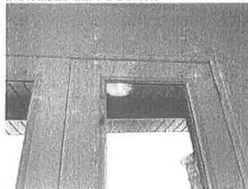
150247 - 3 - FRONT DOORS~SCREW CAPS NOT INSTALLED LEFT DOOR X3
