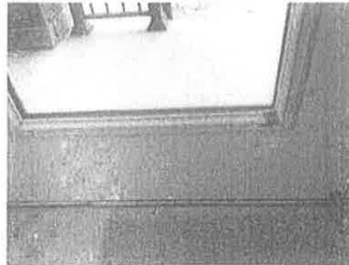
150247 - 1 - FRONT DOORS~SCREW CAPS NOT INSTALLED LEFT DOOR X3
