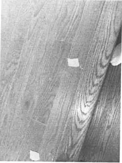
151350 - 1 - FLOORING~CHIP AT 1ST 8TH 9TH 10TH PLANK INFRONT OF NOSING AT STAIRS
