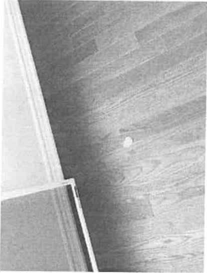
151346 - 1 - FLOORING~CHECKED ON HARDWOOD PLANT IN FRONT OF RIGHT OPERATING WINDOW
