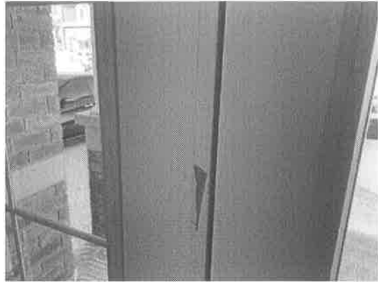
154238 - 2 - FRONT DOORS~CHIPPED ASTRICAL AT MIDDLE FRONT DOOR
