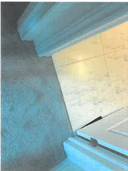
158099 - 1 - FLOORING-ADJUST CARPET SHIM AT THE ENTRANCE TO BATHROOM
