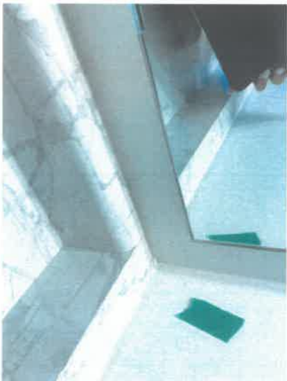
157284 - 1 - NOTE::~CRACK AT RIGHT SIDE SPLASH.
