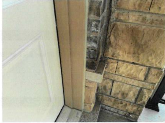
158253 - 2 - PORCH~MISSING MORTAR AT SILL RIGHT AND LEFT SIDE
