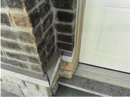
158253 - 1 - PORCH~MISSING MORTAR AT SILL RIGHT AND LEFT SIDE
