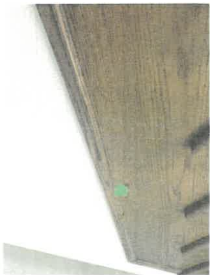
159036 - 2 - STAIRS~CRACK ON OUTSIDE TRIM AT STRINGER AT STAIRS
