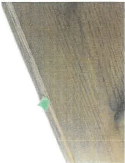
159036 - 1 - STAIRS~CRACK ON OUTSIDE TRIM AT STRINGER AT STAIRS
