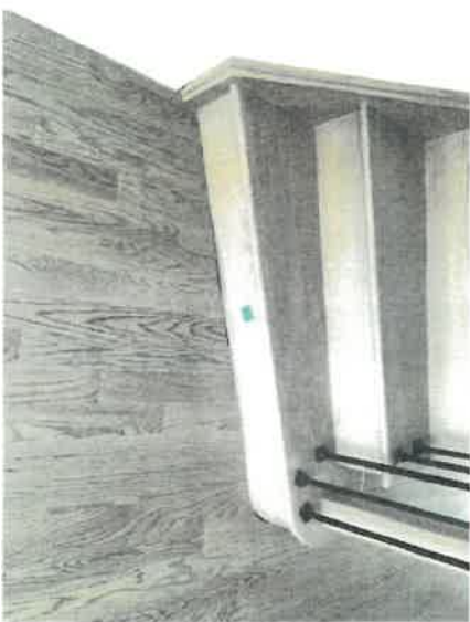
160577 - 1 - STAIRS-TRIM NOT INSTALLED BELOW STRINGER AT MAIN FLOOR STAIRS
