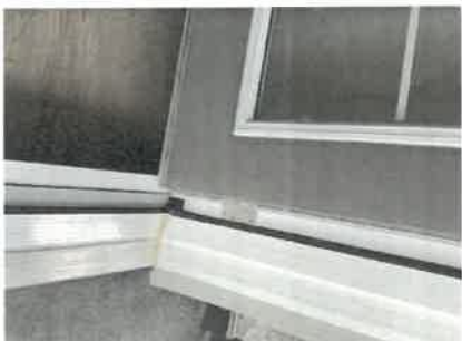
160789 - 1 - WINDOWS-ADJUST SCREEN DOOR AND WEATHER STRIP AT BALCONY DOOR ABOVE FRONT PORCH
