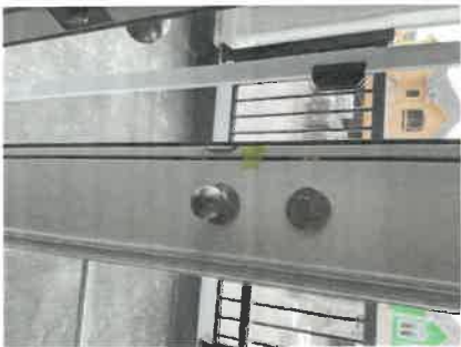
160788 - 1 - TRIM-GAP AT FIXED DOOR AND ASTRICAL AT BALCONY ABOVE PORCH
