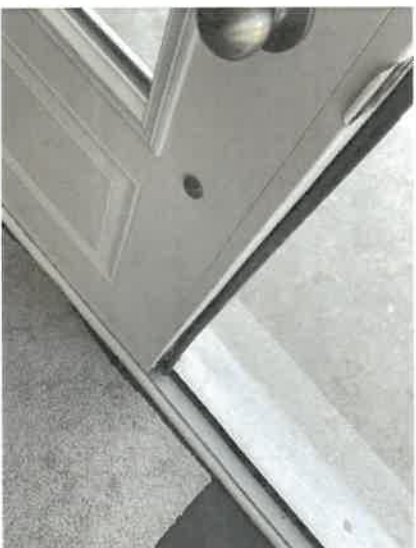
160798 - 1 - FRONT DOORS-SECURE WEATHERSTRIP AT FRONT DOOR
