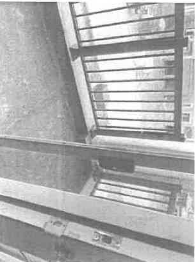
160789 - 2 - WINDOWS~ADJUST SCREEN DOOR AND WEATHER STRIP AT BALCONY DOOR ABOVE FRONT PORCH
