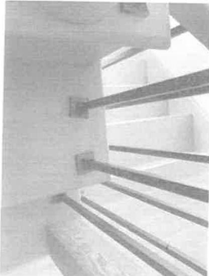
164579 - 2 - STAIRS~REMOVE PAINT FROM PICKETS THROUGHOUT
