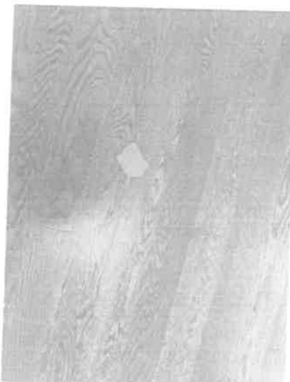
161077 - 1 - FLOORING~CHIPS ON HARDWOOD MARKED WITH GREEN TAPE
