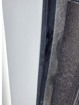
159031 - 1 - IMG-20230702-WA0005 - Flashing loose at left side OF GARAGE DOOR
