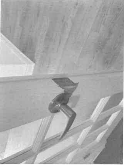
168018 - 1 - NOTE::~ADJUST LOCK , STICKING OUT AT DEN
