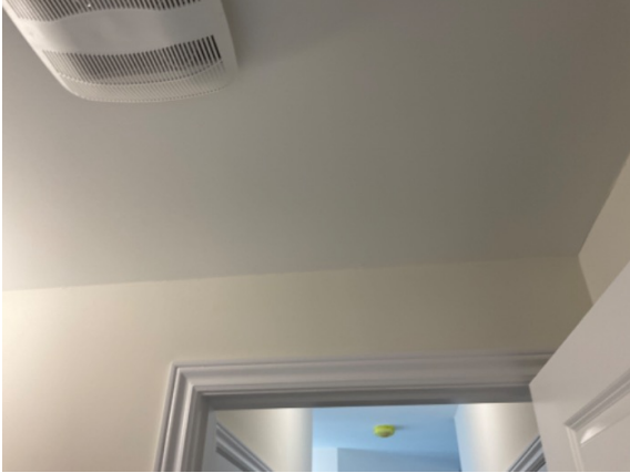
164524 - 1 - NOTE:~ROUGH DRYWALL AT CORNERS ABOVE DOOR
