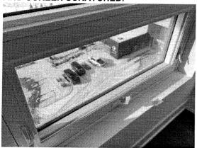
171361 - 2 - NOTE:~MISSING WINDOW CRANK AND SCREEN SCRATCHED.
