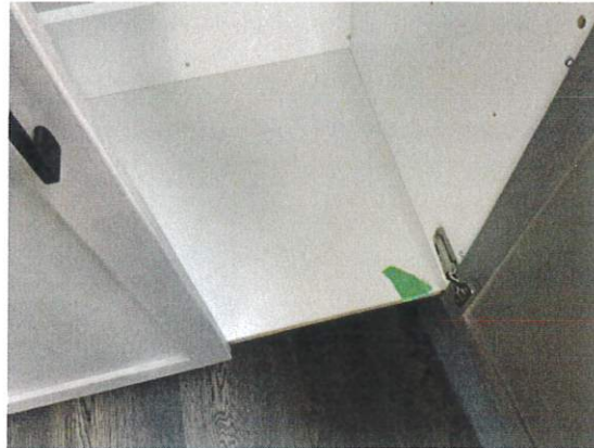
163254 - 1 - CABINETS~CHIP AT BOTTOM GABLE RIGHT OF SINK AT CABINET.
