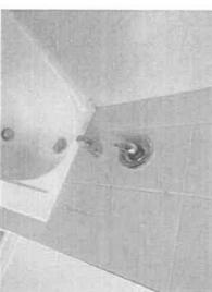
line was damaged or missing at areas on the air-conditioning suction (large, insulated) 180153 - 1 - 80000c96-c4e6-4c99-989e-d45a590d1753 - REFRIGERANT LINES:Insulation
