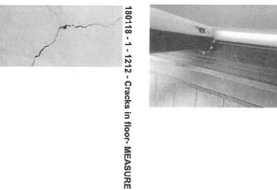
180116 - 1 - 1212 - Water comes in from bottom of window which leaks on hardwood floor which has a few cracks. Rust mark in middle of window on the inside between glass-PHOTO
