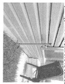
180140 - 1 - d00d273a-9327-49bf-aa28-6d664535270c - Windows in the home had inadequate clearance from grade.- SVC MEASURE
