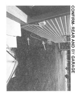
that will route runoff from precipitation toward the foundation as a result of backfill settlement- SVC 180146 - 2 -6f0fa156-da6c-47fe-8099-23ddc962115b - he INSPECT AND CONFIRM- REAR AND BY GARAGE building had areas of neutral or negative drainage
