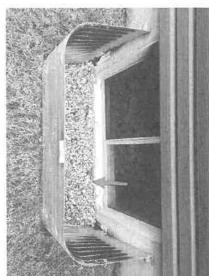
aa28-6d664535270c - Windows in the home had inadequate clearance from grade.- SVC MEASURE IN SPRING TIME
