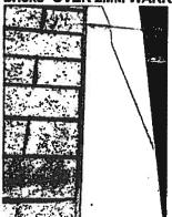
183525 - 1 - 20250623\_145108\_resized - Around the front door the mortar has shrunk away from the bricks. Also there is mortar residue smeared around the large blocks that surround the front door:- OVER 2MM WARRANTED 2YEARS,
